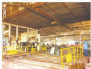
Seven Tank Phosphating System
